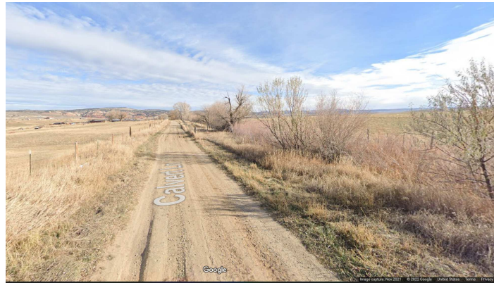
Figure 1.5. View of Yankee/Calvert Lane lateral canal on right side of road which experiences high seepage loss resulting in undesirable vegetation growth along the canal.
